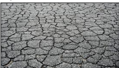
Fig. 3. Alligator Cracking
