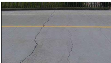
Fig. 2. Transverse Cracking
