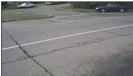
Fig. 1. Reflecting Cracking
