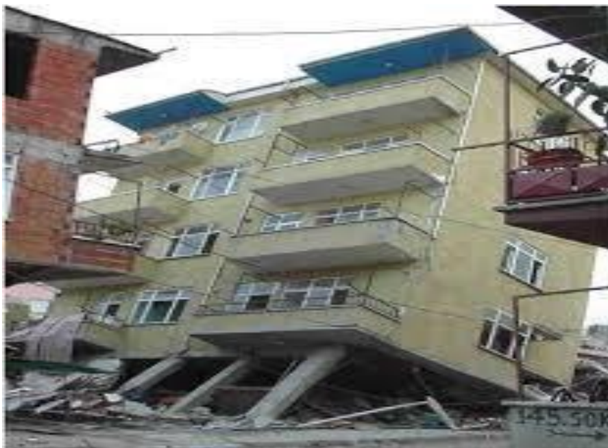
Fig.1 Collapse of a building with soft storey
