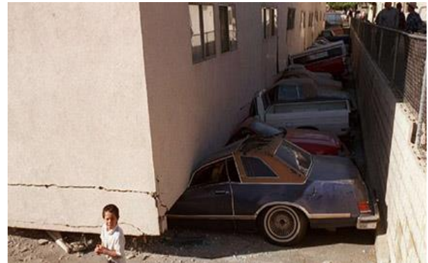
Figure 1: Soft storey building failure.
