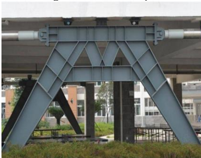
Fig 1.3 Viscous damper
