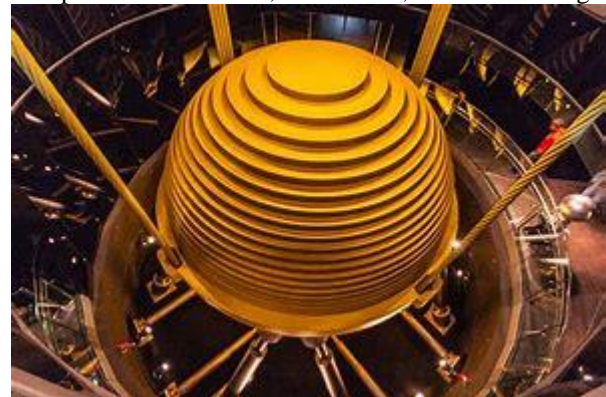
Fig 1.1 Tuned Mass Damper
