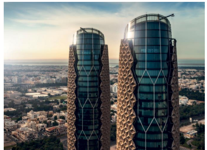
Fig 1. Example of hexagrid structure
