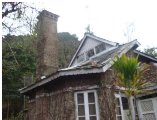
Image 2: Exterior view of the house
