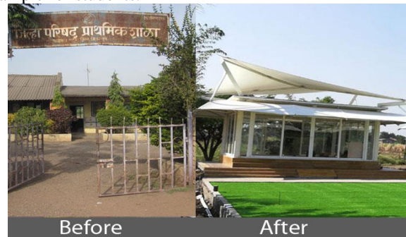
FIG 7: -- Zero Energy School Wablewadi, Dist. Pune
