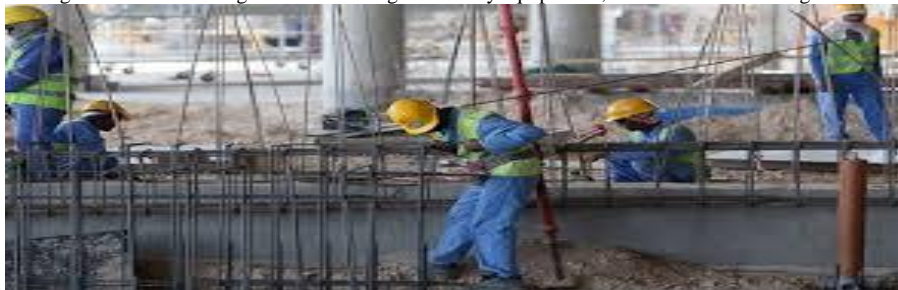
Figure: Picture showing workers at construction site.
