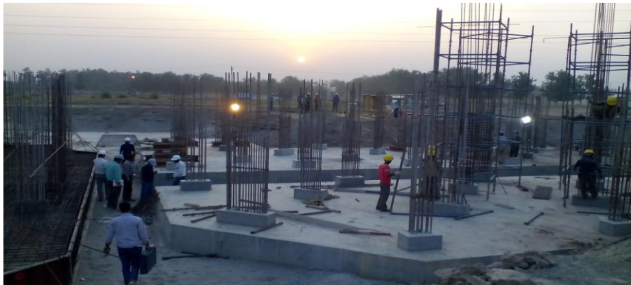
Figure: Picture showing safety at construction sites.
