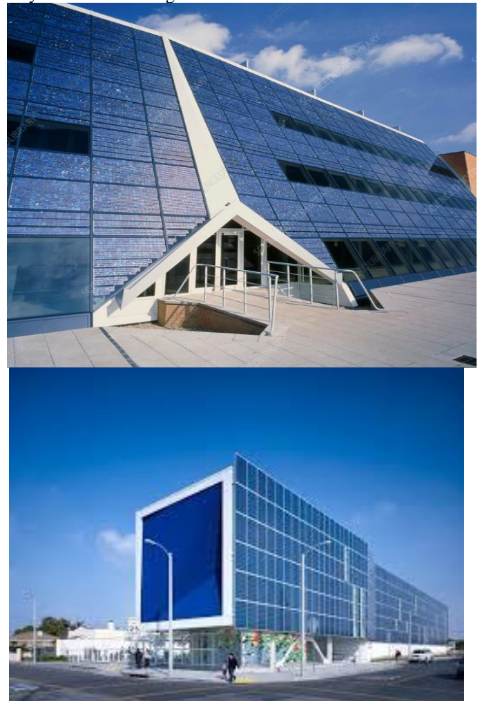
Fig. 1. integrates solar cell in façade design through environmental graphic aspects
