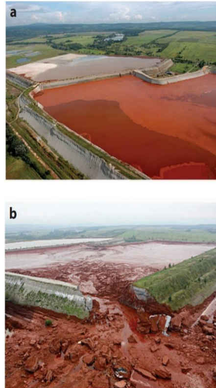
Figure 2: (a) red mud tailing in Hungary and (b) 2010 dam failure (Boger 2013)
