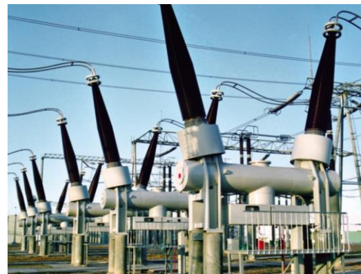
Fig. 1. A Dead Tank Circuit Breaker
