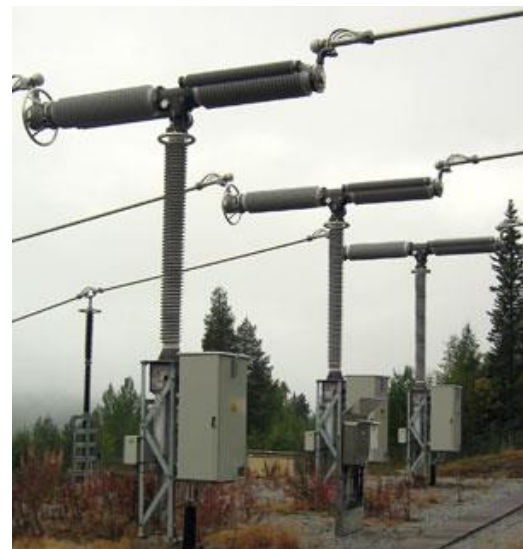
Fig. 2. A Live Tank Circuit Breaker
