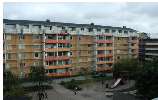
Figure 2.2 Husby project after reconstruction
