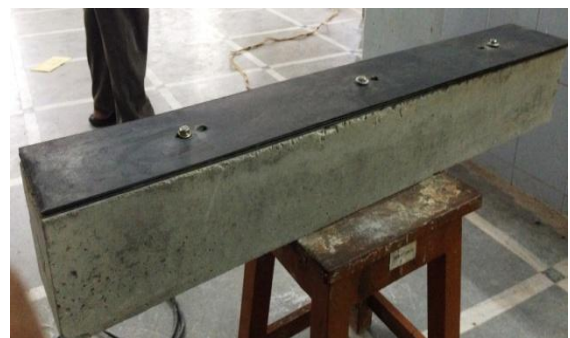
Fig 1 RCC Beam retrofitted with MS plates
