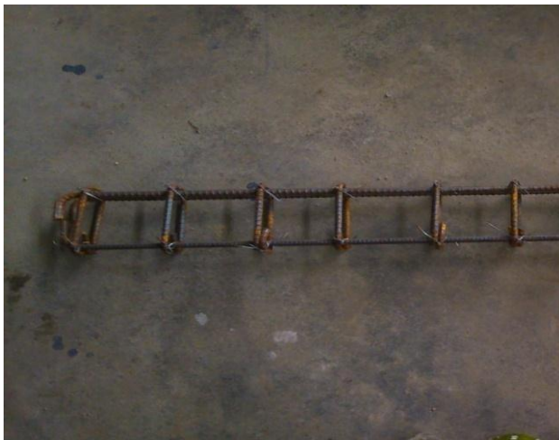
Fig.1. Cage of Beam
