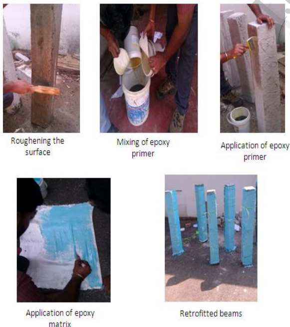
Fig 3 Retrofitting of beams
