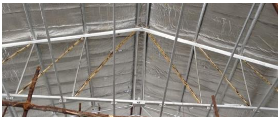
Fig 3 Inclined braces welded with 16mm and 20mm dia. Bars
