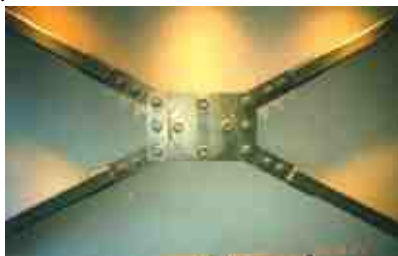
Fig. 2. Friction Damper in tension-only cross brace [21]
