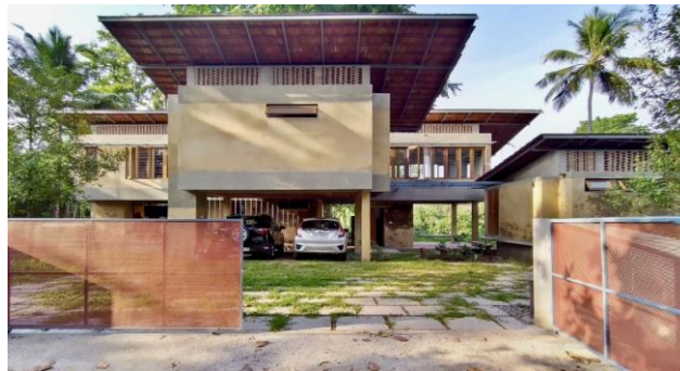
Fig.2. View of The Garden Terrace House from the entry gate. The simple rectangular volumes with voids on the ground floor acting as water discharge spaces, to combat flooding, are visible.
