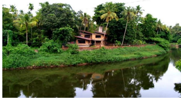
Fig.1. View of The Garden Terrace House from the bridge across Kurumali river. Design compromises like the large windows facing west affords excellent views of the river but increases solar heat gain.
