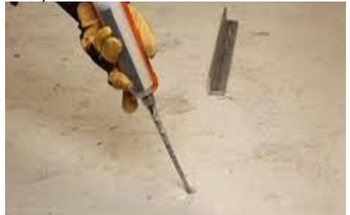
Fig. Resin Injection
