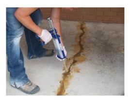
Routing and sealing: This method, the crack is made wider at the surface with a saw or grinder, and then the groove is filled with a flexible sealant.
