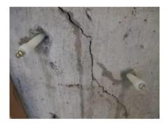
Gravity filling: Low viscosity monomers and resins can be used to seal cracks with surface widths of 0.001 to 0.08 in. by gravity filling. High molecular weight methacrylates, urethanes, and some low viscosity epoxies have been used successfully.
