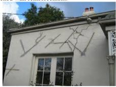
• **Drilling and Plugging:** This technique is only applicable when cracks run in reasonable straight lines and are accessible
