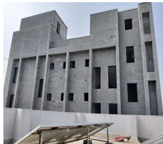
Fig. 1. Construction near PV power plant
