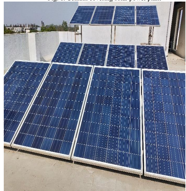
Fig. 7. Solar power plant after cleaning
