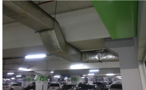
Figure6. The more fluctuation in channels for air - conditioning
