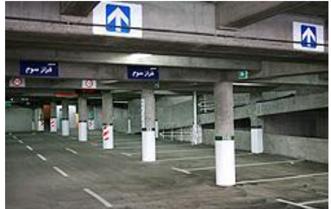
Figure 4. Normal beam in parking area
