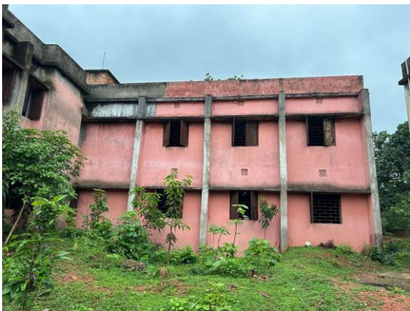
Fig. 2. External elevation of the hostel showing weathering, staining and vegetation (photograph supplied by the author; date and orientation not recorded)
