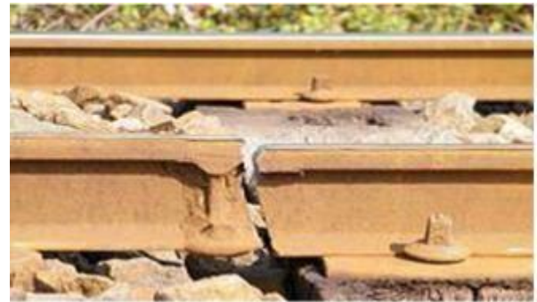
Figure. 1. Railway crack on track
