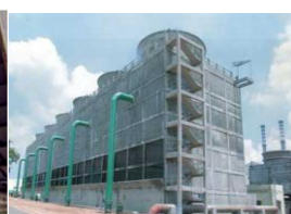
Figure-5 RCC made Cooling Tower
