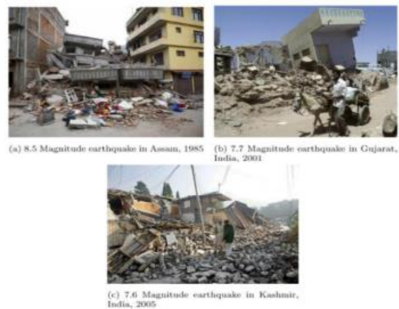
Fig 1: Destruction caused by an earthquake in recent years.
