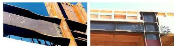
Figure 2. Application of Reduced Beam Section (RBS) Connection
