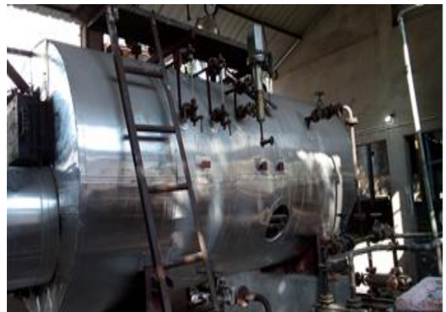
Fig. 2. Boiler Section with water level gauge
