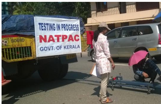
Fig. 2. Deflection measurement using Benkelman Beam
