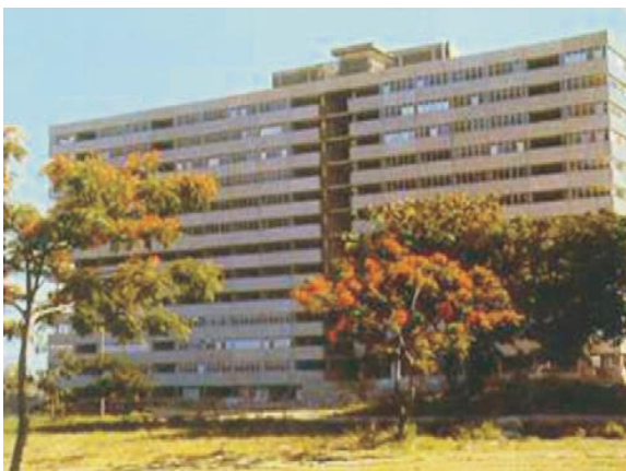
Figure 1: A typical precast slab-column building.
