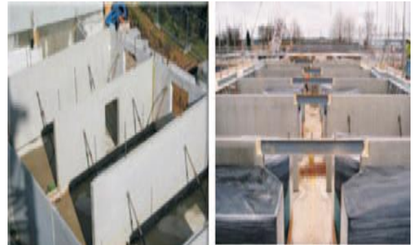
Figure 7: Use of precast concrete in hotel construction
