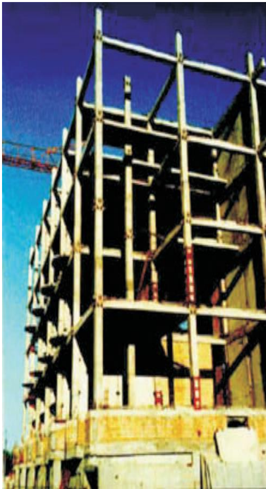
Figure 6: Seismic strengthening of precast columns with steel straps
