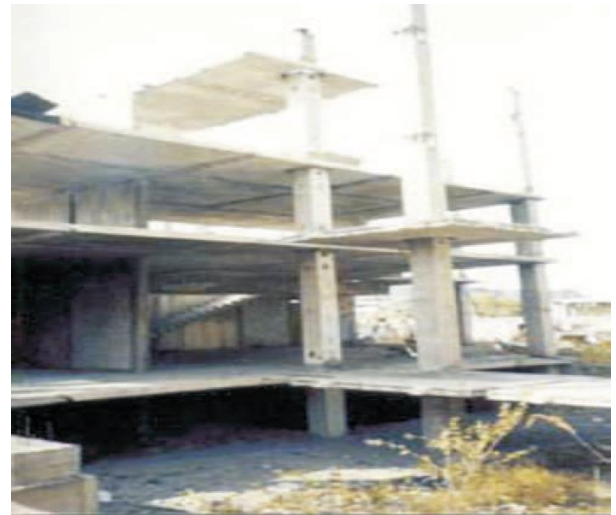
Figure 5: A lift-slab building under construction
