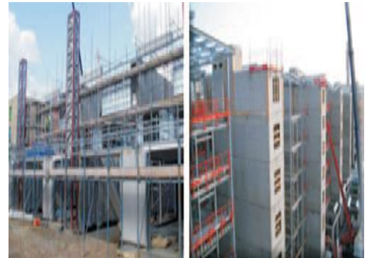
Figure 9: Use of Precast concrete technology in apartment construction
