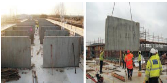
Figure 2b: Cross Wall construction
