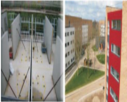
Figure 8: Use of precast concrete in hostel construction
