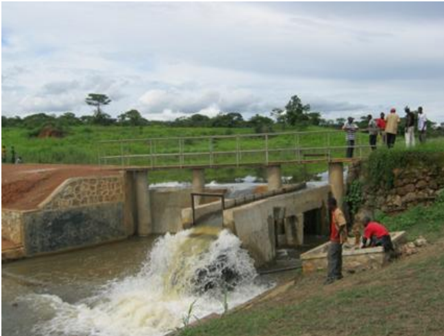
Fig 1a; A recently rehabilitated spillway of St Mary's dam before being clogged and damaged. Note that initially the dam had four pillars. December 2011. (Photo: Mumba Kolala).
