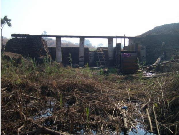
Spillway before the initial rehabilitation works July 2010. (Photo: Mumba Kolala).
