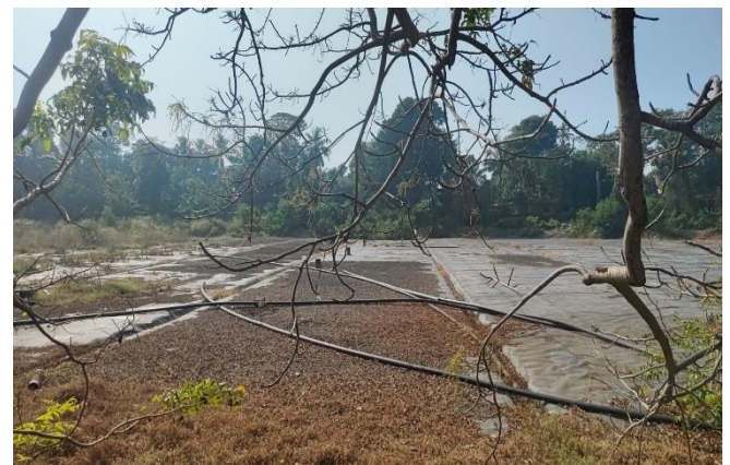
Fig. 1. Kureepuzha Dumpsite after Biomining
