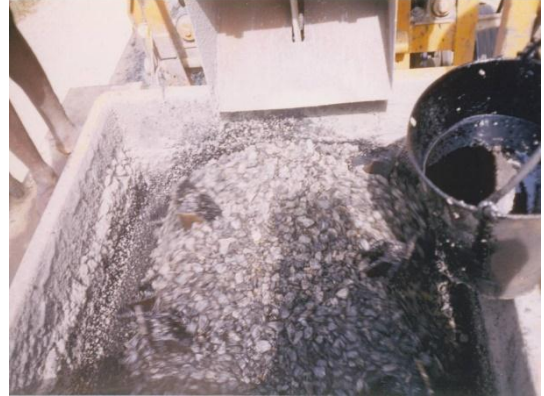
FIG 10: Bitumen being mixed with plastic coated aggregates.
