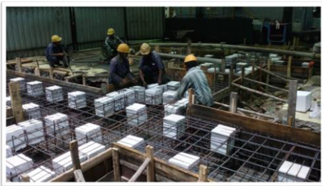
Fig 1. Use of Thermocole box as pockets formwork
