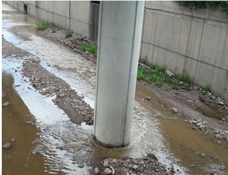
Figure 2. Light scour on a bridge pier after raining.
