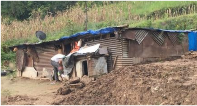
A temporary shelter after earthquake build by people
