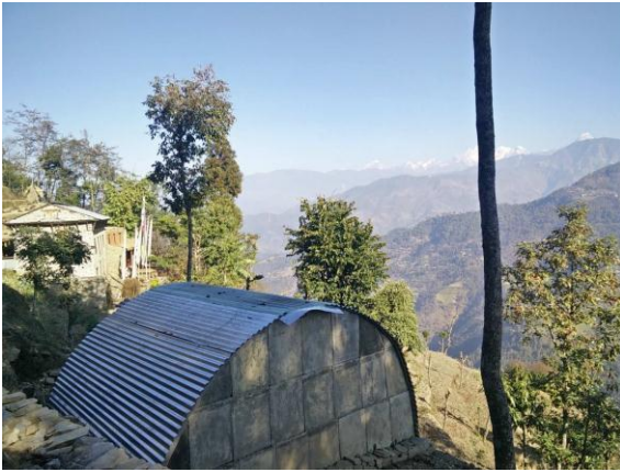
Shelter provided of mud & GI sheet as an immediate relief
