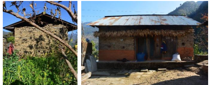
Photographs of the houses showing the roof and entrance of the traditional houses in Ratankot
