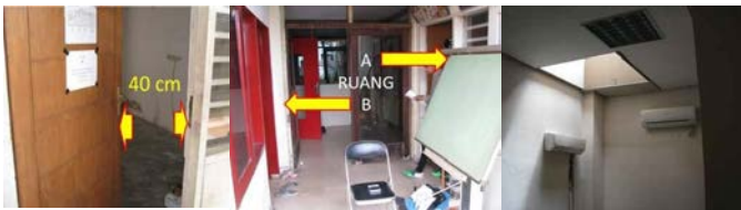
Fig. 1. (Left) The Door Opening Distance For Each Modified Room To Maintain The Existing Air Velocity (v) From The Outdoor; (Center) The Corridor Outside the Modified Rooms; (Right) The Additional Void Built in the Room A
