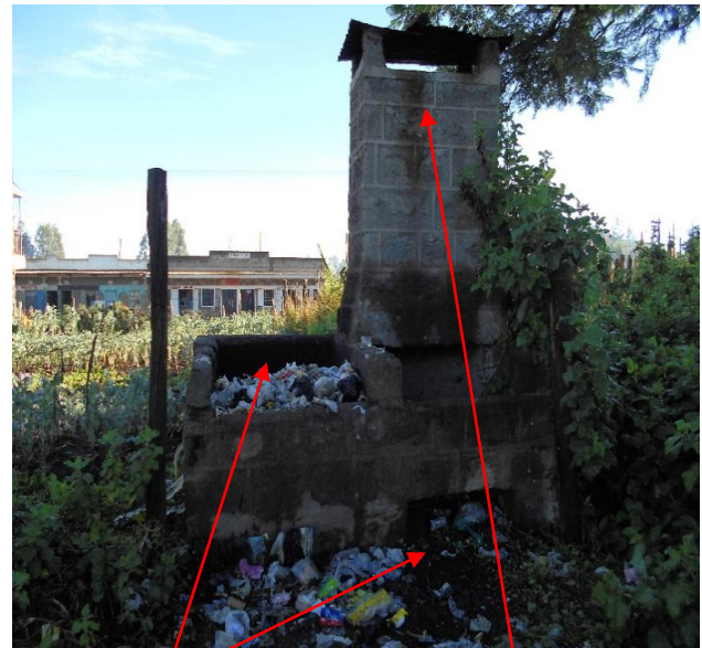
Open-Waste Burning Outside Incinerator Poorly Designed Incinerator
