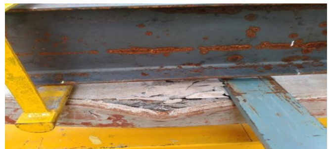
Plate 2. Separation of concrete and steel
