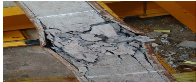
Plate 1. Buckling of steel in compression zone
