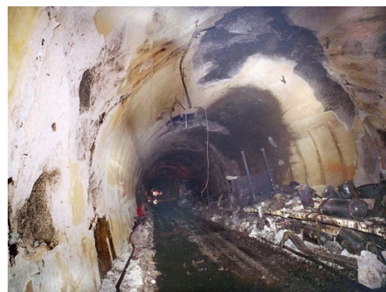
Fig. 4: Spalling due to fire in the Mont Blanc Tunnel fire (1999)
