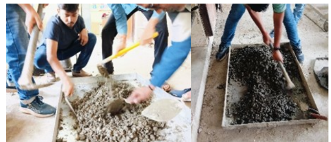
Fig. 1. Batching of materials
