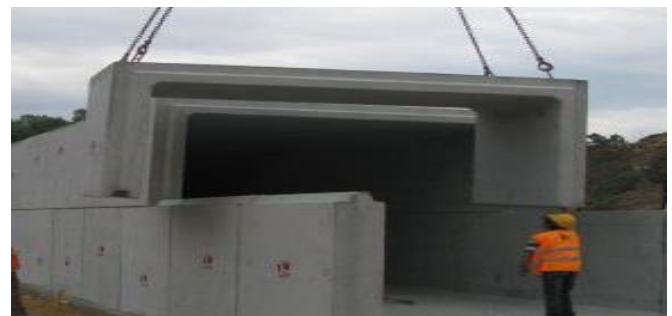
Figure No. 01 – Culvert with Hinge Joint at Mid of Wall
