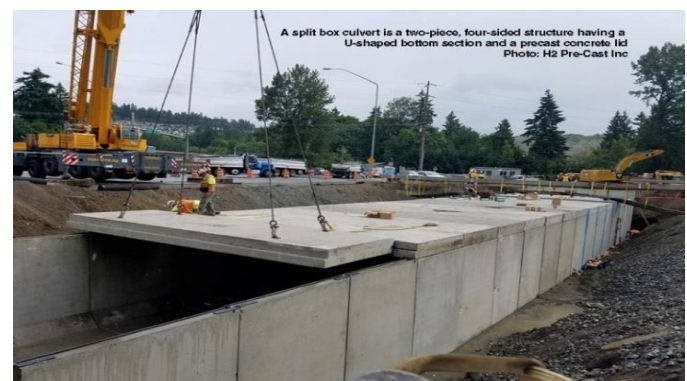
Figure No. 02 – Culvert with Hinge Joint at Top
