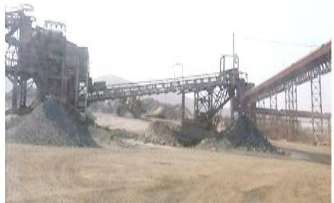
Figure 5 Disposed LD & HMDS slag at slag yard
