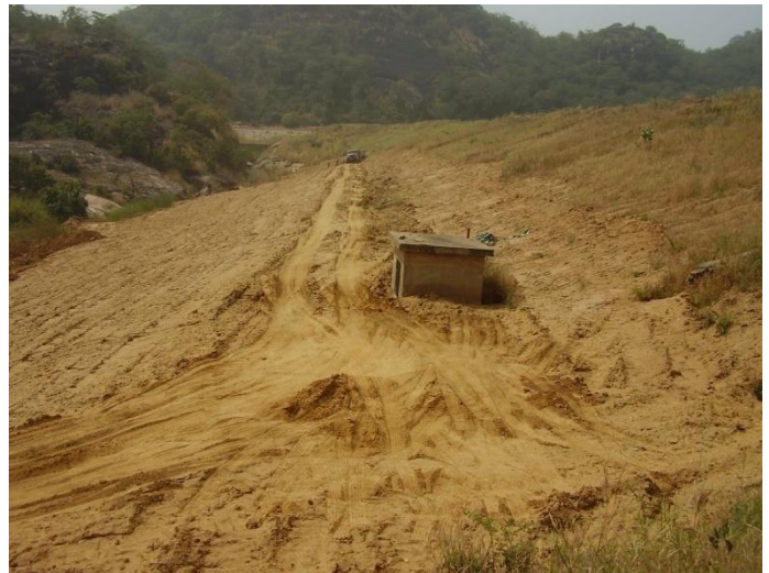
Figure 13; Rehabilitation work in progress at Waya Dam in Bauchi after failure
