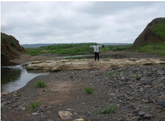
Figure 16; Complete Failure of Cham Dam in Gombe
