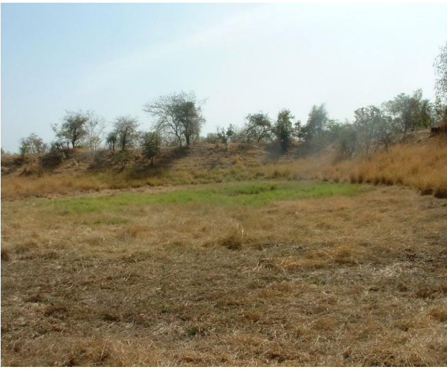
Figure 8; The reservoir of SB/GR Dam 2 remains empty
