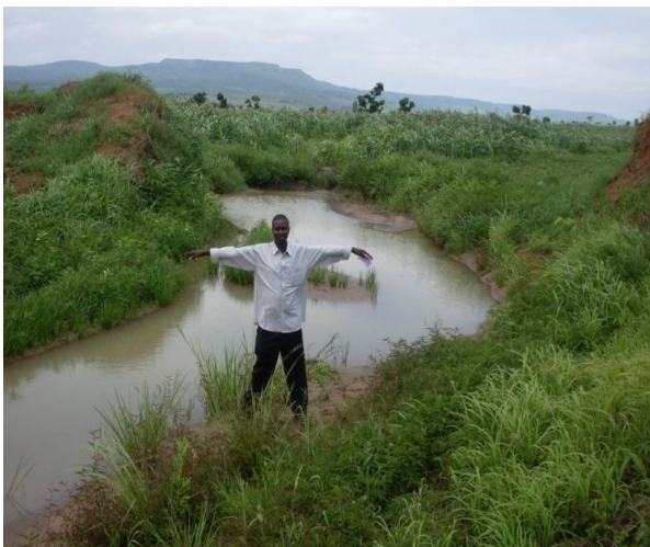
Figure 6; Complete Failure of Bambam Dam in Gombe
