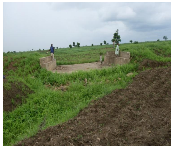
Figure 7; Bambam Dam Spillway
