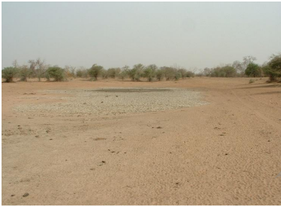
Figure 4; N/G G Reserve Dam 1 Dalehi Silted up
