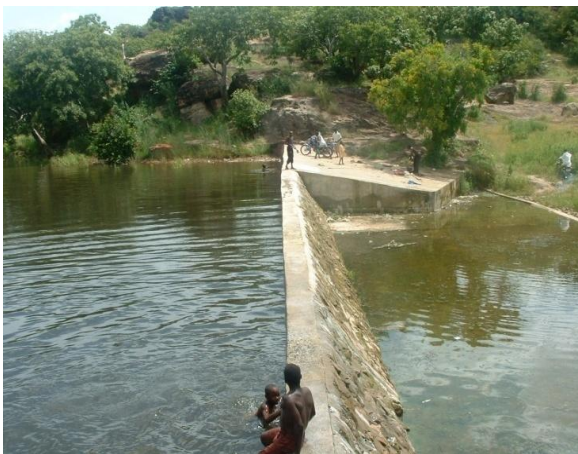
Figure 10; Girei Dam reservoir about to spill and rehabilitated Spillway
