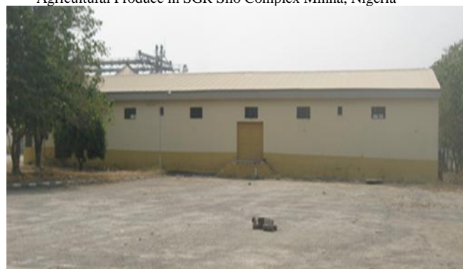
Plate 2: Exterior View of Specialised Warehouse for Storage of Gari and other Agricultural Produce in SGR Silo Complex Minna, Nigeria.
