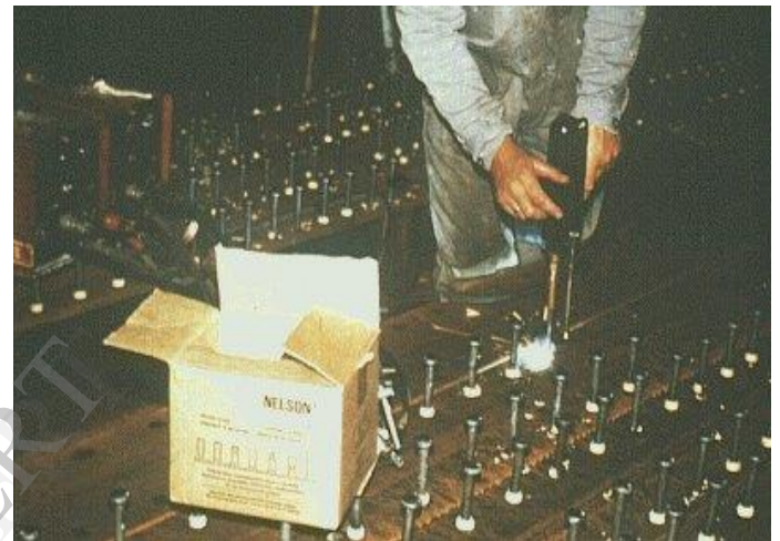
Fig. 4 Semi-Automatically Welded Headed Studs
