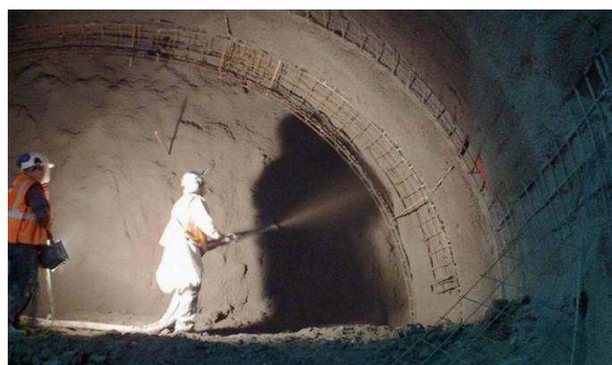
Fig. 17 Face Sealing Shotcrete
