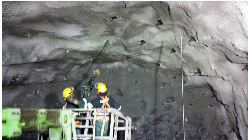
Fig.30 Rock Bolt Installation
