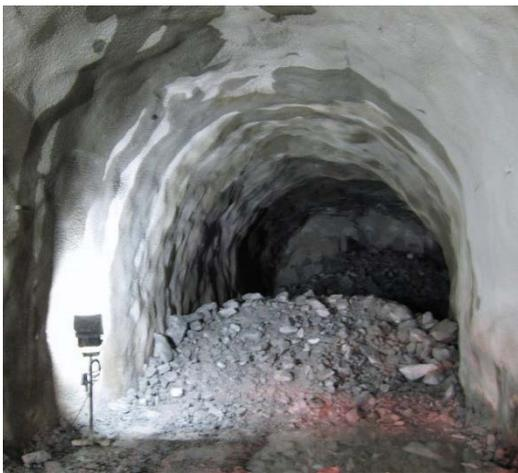
Fig. 12 Muck in the tunnel
