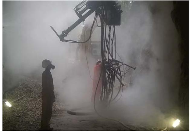
Fig. 11 defuming of gases after blasting from tunnel
