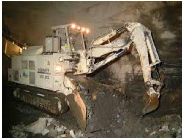
Fig.13 Hagg Loader used in removal of muck
