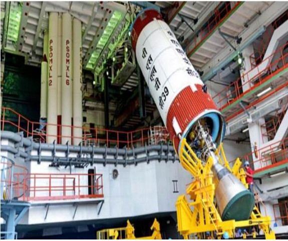
Fig: PSLV-C39 Liquid Stage at the Vehicle Assembly Building during Vehicle Integration
