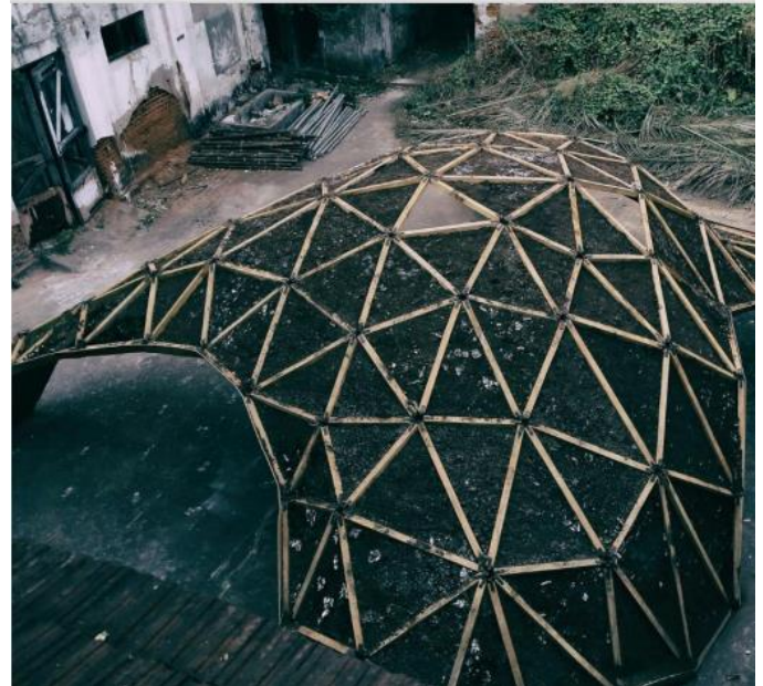
Figure 11: Top View of The Structure.
