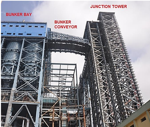
Figure 1 Adjacent component of Junction tower (Courtesy: BHEC)
